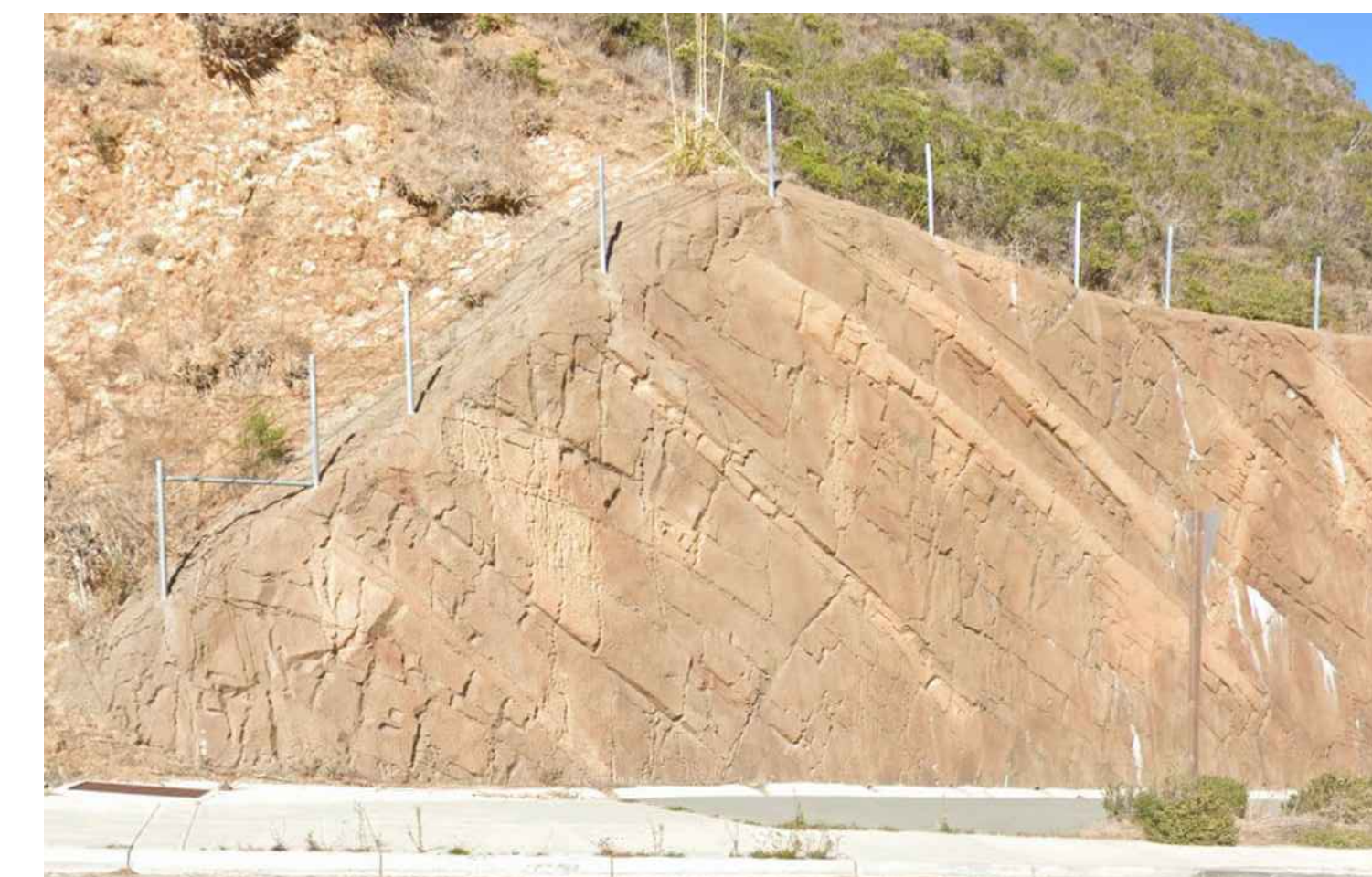
G RETAINING WALL SCULPTED SHOTCRETE
